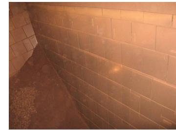
Same Laminite® Rubbadex wear plates in use
